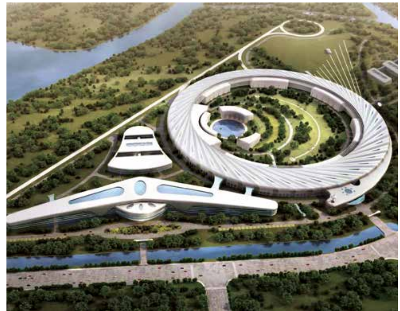
The High Energy Photon Source (HEPS) will be built in China.
